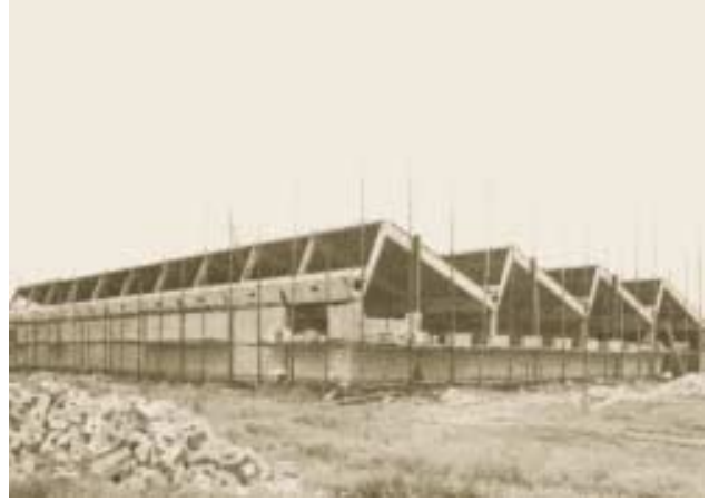
Construction of the new factory at Hemmingen.
